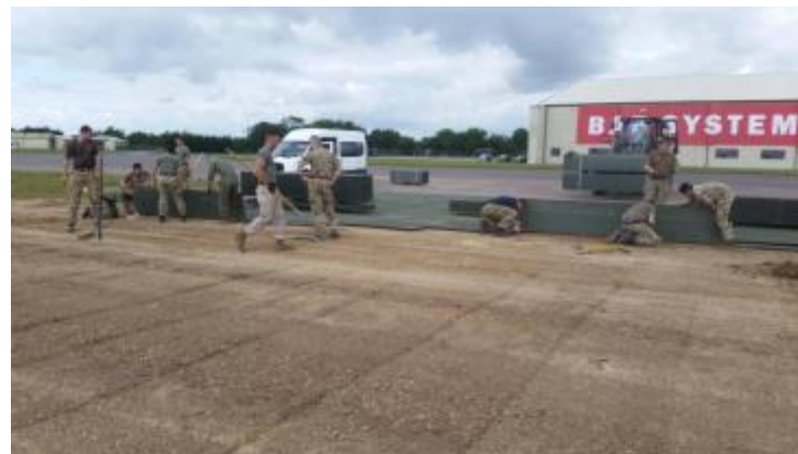
Marine Wing Support Squadron -273 and British Army engineers install a VTOL pad in support of the F-35B at Royal International Air Tattoo, summer 2016
